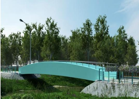
**MOBISTEK all-composite bridge span** is made of polymer composite materials by vacuum infusion.
