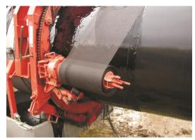
**SST-B** *TRANSET* **fiberglass reinforcing mesh** is a mesh of glass fibers, which is impregnated with a compound based on bituminous or bitumen-polymer primers.
